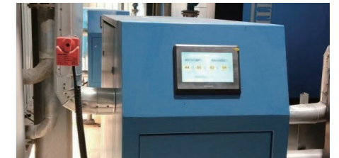
Waste Heat Recovery Transformation of Air Compressor
