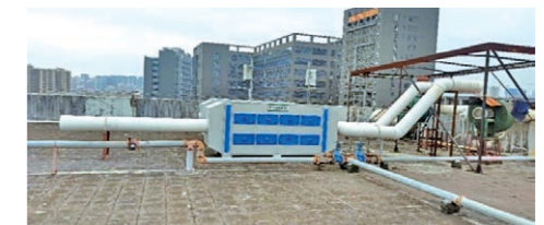
Installation of Activated Carbon Filter Box on Rooftop of the Factory
